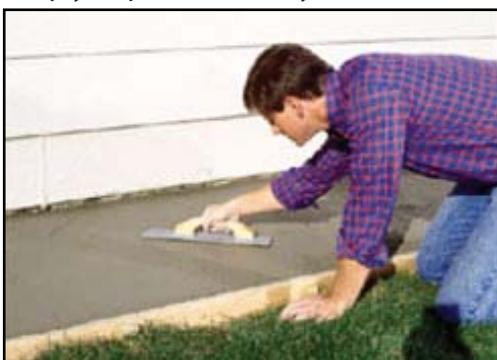
After the bleed water is all gone you can get out your steel finishing trowel and put on the final touches. You will notice the steel trowel is not perfectly flat. That is done so that when you trowel you will be more prone to lift the leading edge slightly avoiding digging into the concrete.
